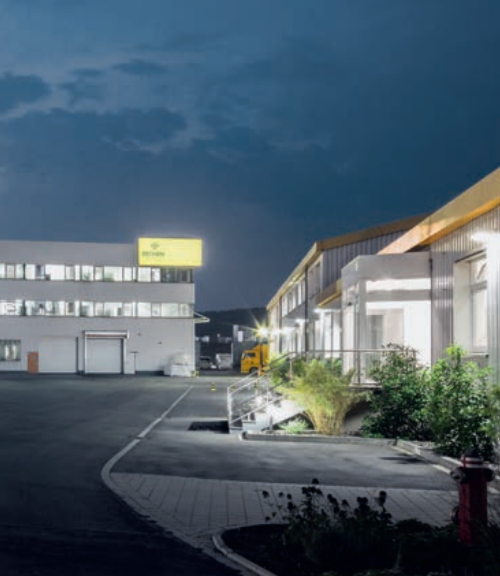
BECHER headquarters in Hagen, Germany
